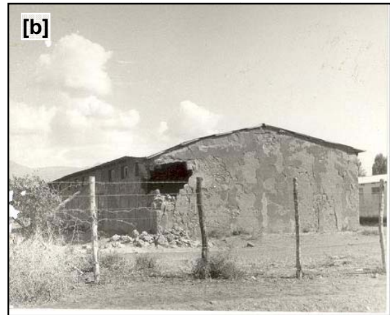
Figure 5 (a) Damage to Wetera Abo Church in Wondo Genet (1983 earthquake). (b) Damage to Arba Minch Kebele Warehouse (1987 Earthquake Swarm, masonry building. Damage seems to be caused by biaxial bending at corner of building). (Photo source: Dr. Laike Mariam Asfaw - private communications).
