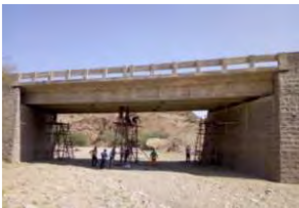
Figure 13 Set-up for truck loading test
