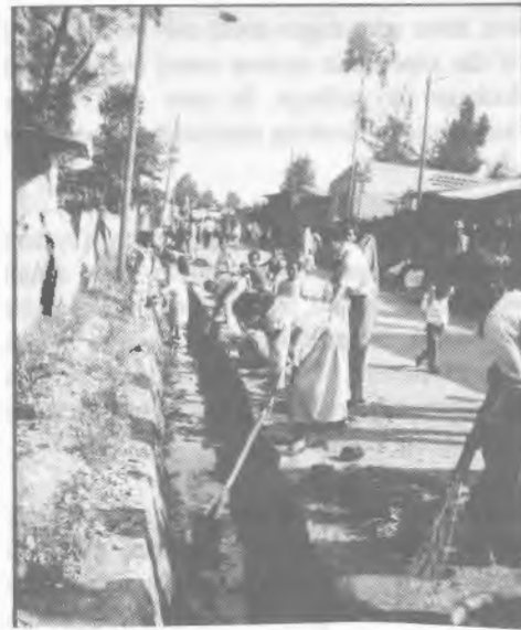
Plate 3: Cleaning open drains (Note the use of shovels & the pile of garbage at the edges)
