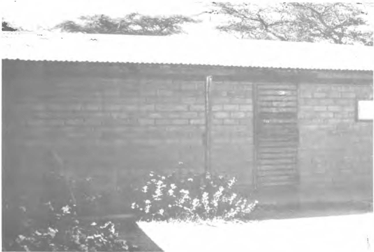
Fig. 5 School Constructed of Soil-Cement Mixture Block
