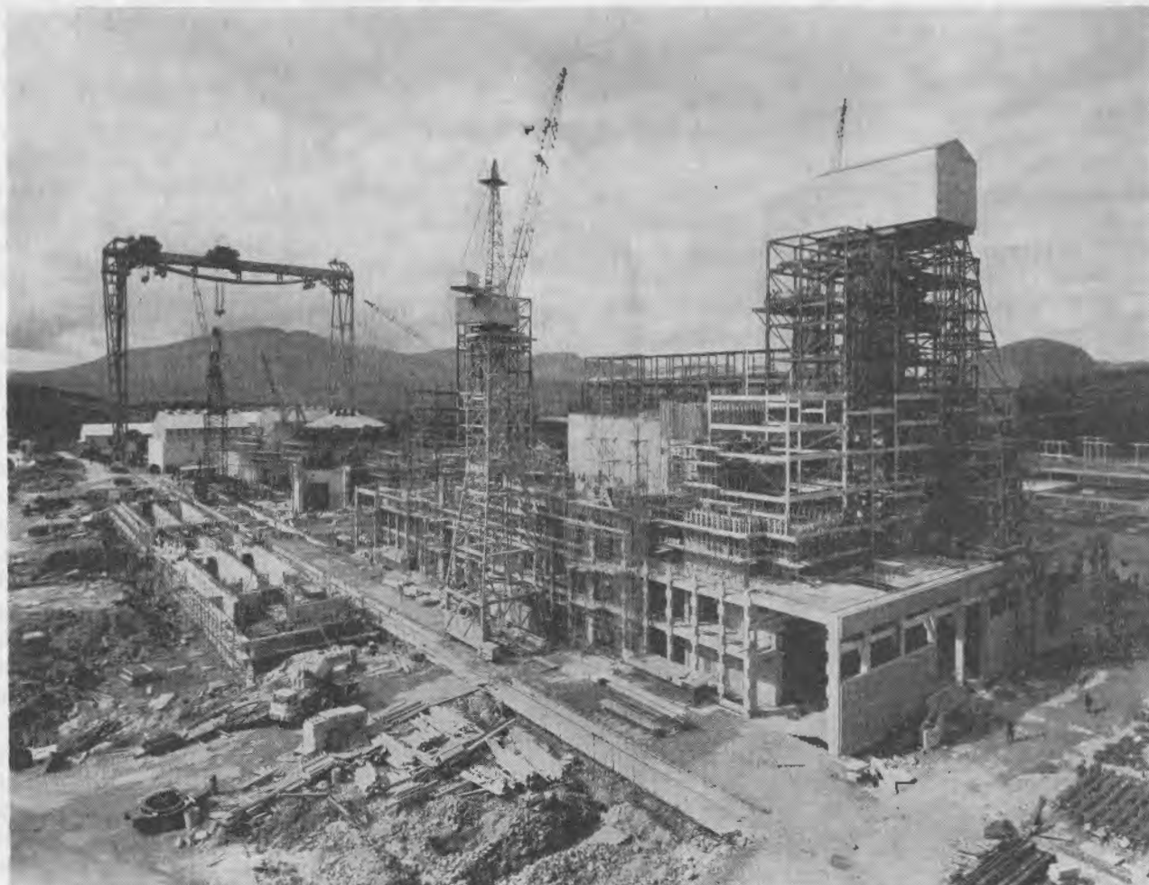
Fig. 2 — The C.E.G.B. Nuclear power Station at Trawfyndd during the constructional period
