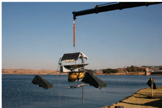
Figure 9 Deployment of a SolarBee® laminar flow pumping unit in Rietvlei Dam during 2008
