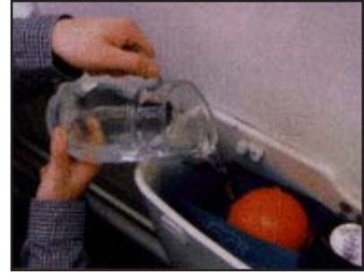
3. Flush toilet in normal manner whilst simultaneously pouring about 4 ℓ of water into Hippo
