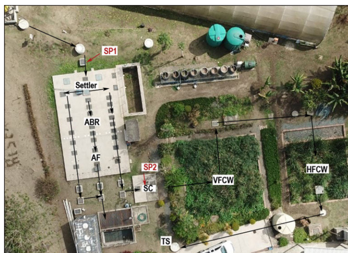
Figure 1. Aerial view of the Newlands Mashu decentralised wastewater treatment system (taken September 2019) ABR = anaerobic baffled reactor; AF = anaerobic filter; HFCW = horizontal flow constructed wetland; SC = siphon chamber; TS = trunk sewer; VFCW = vertical flow constructed wetland. Black arrows denote the direction of flow. Flow from Train 1 of the ABR is further treated in a hybrid subsurface flow constructed wetland system.
