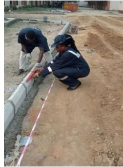
Fig. 3: Center for Wetland and Waste Management Studies During Landscaping
