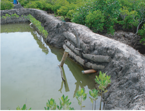
Figure 2. A pond at Majaoni showing the PVC standpipe to drain the pond and the overflow pipe that allowed water exchange at spring high tides and maintained the water level.
