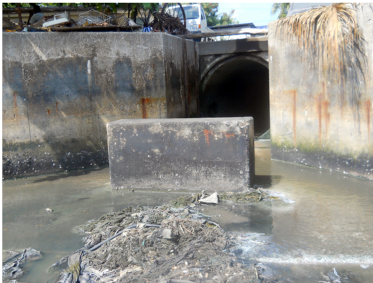
Figure 2. Sewage outlet in Bwawani area, from which waste discharges into coastal waters.
