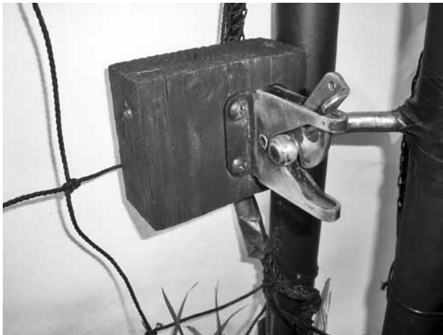
Figure 3. Close-up of gate latch. (photograph: David R. Barber)
