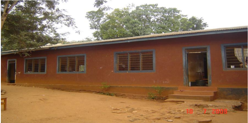
Photo1: Classrooms Constructed at the Mlali Primary School
