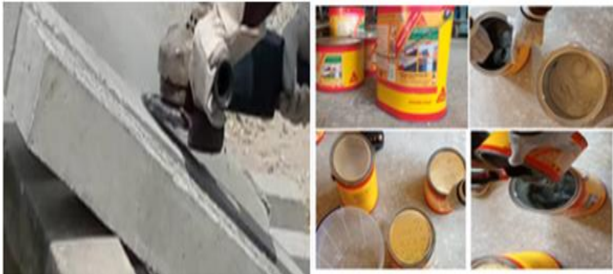
Figure. 2: Beam surface treatment and Epoxy Resin
