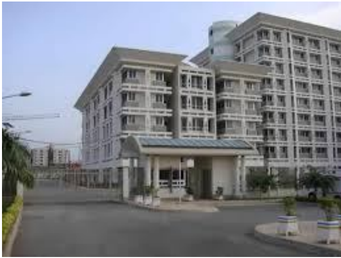
Plate 1: A typical multi-storey office property in Wuse, Abuja
