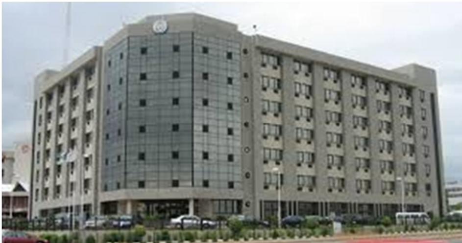
Plate 2: A typical multi-storey office property in Wuse, Abuja
