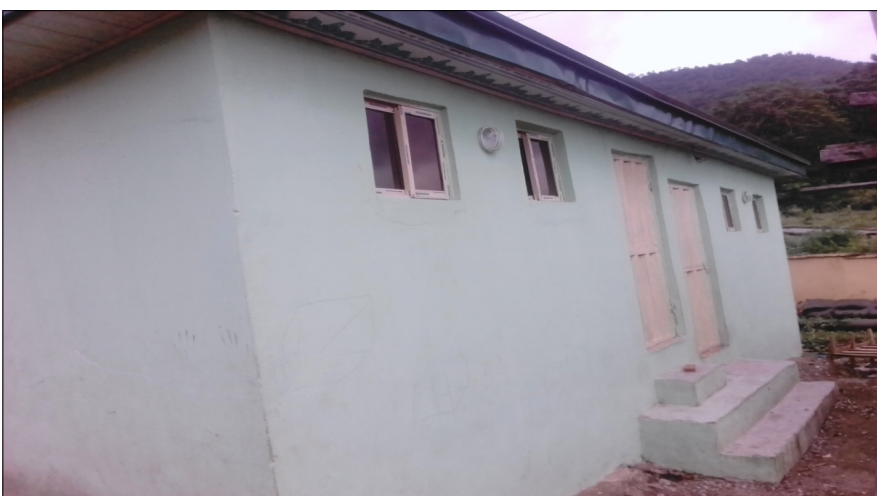
Figure 3: A yet-to-be-commissioned Federal Government-provided 6-water closet toilet facility in Kabawa
