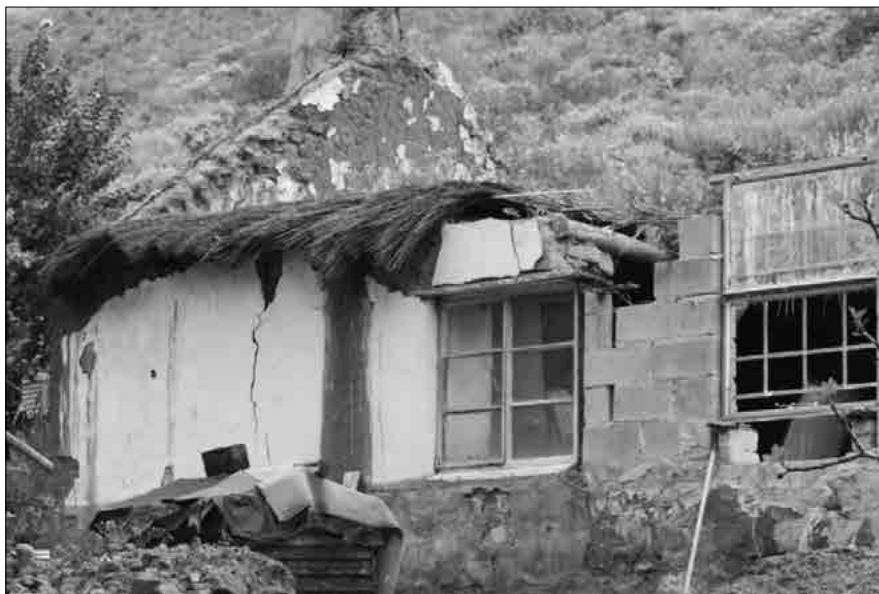
Figure 2: A dilapidated thatch cottage along the main road in the Kerk Straat precinct Source: Image by author, 2016
