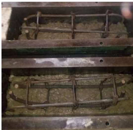
Figure 8: Casting of Steel reinforced concrete beam specimens.
