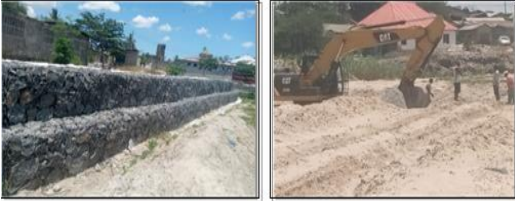
(a) A wall built along the banks of Msimbazi river
