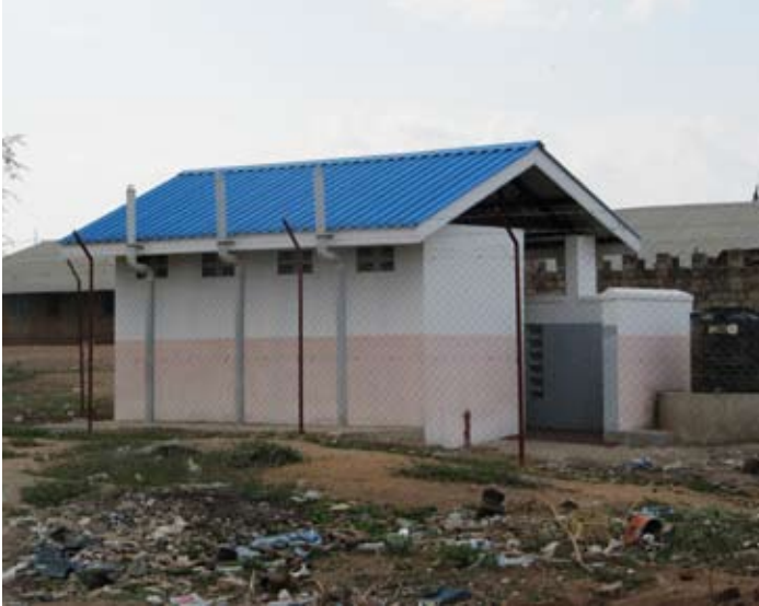
Figure 2. A ventilated pit latrine in Buluk area of Juba, South Sudan (credit Victor Vuni Joseph)
