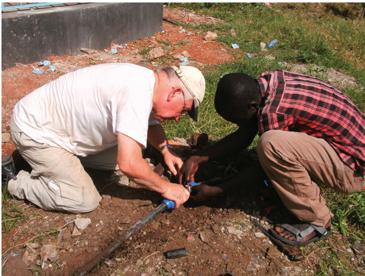
Figure 2. Fixing the plumbing (Nancy MacKeith)
