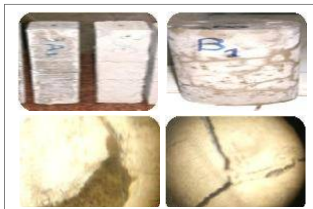
Figure.7: Cracks, checking cracks, gel exudation and discoloration faces in the cylinder and prismatic samples with (B) concrete during 6 storage months (M24X).
