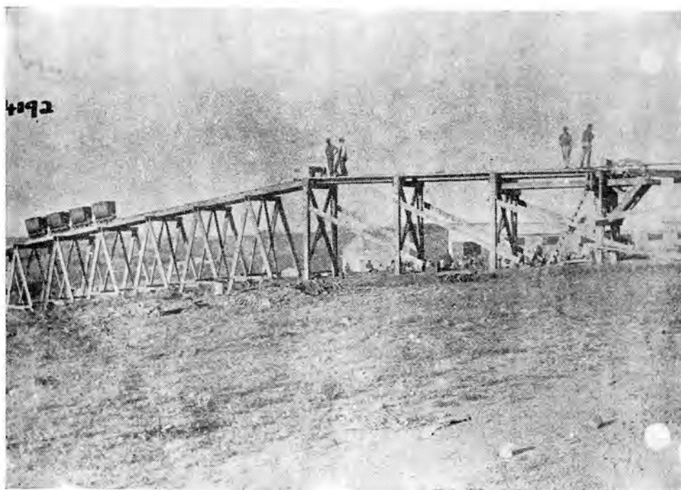
The commencement of the construction activities.
