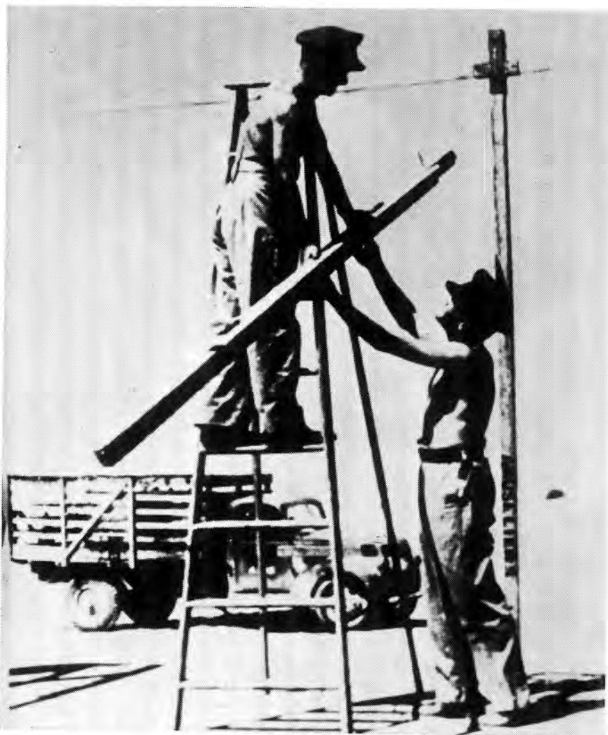
Building a stage: the first step
