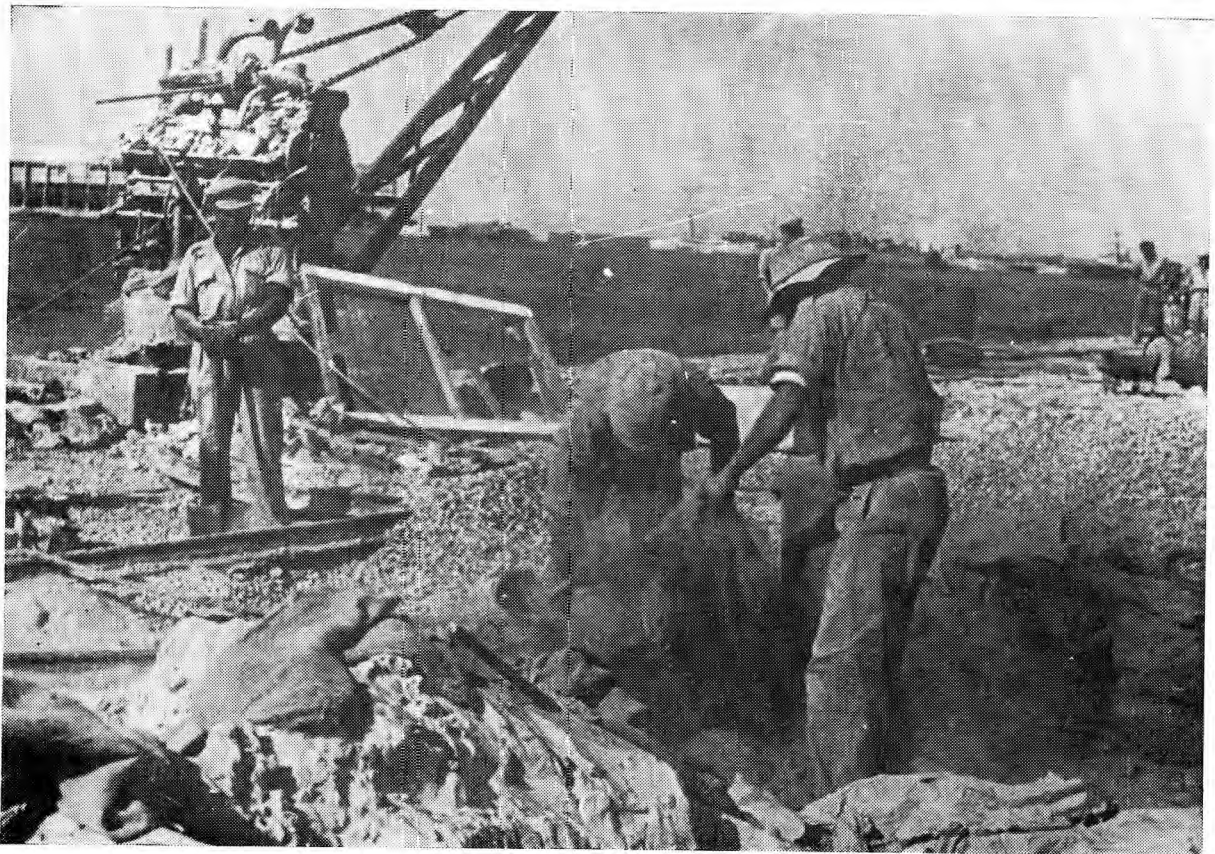
Sappers strengthening the coastal defences.
