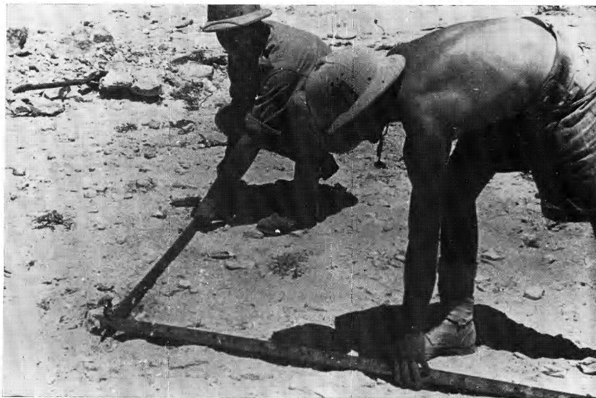
Sappers marking out blasting positions.
