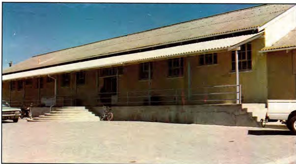
This building was occupied by the CPGI and served as the main shop on Robben Island from 1 February 1949. (With permission of the Department of Correctional Services)
