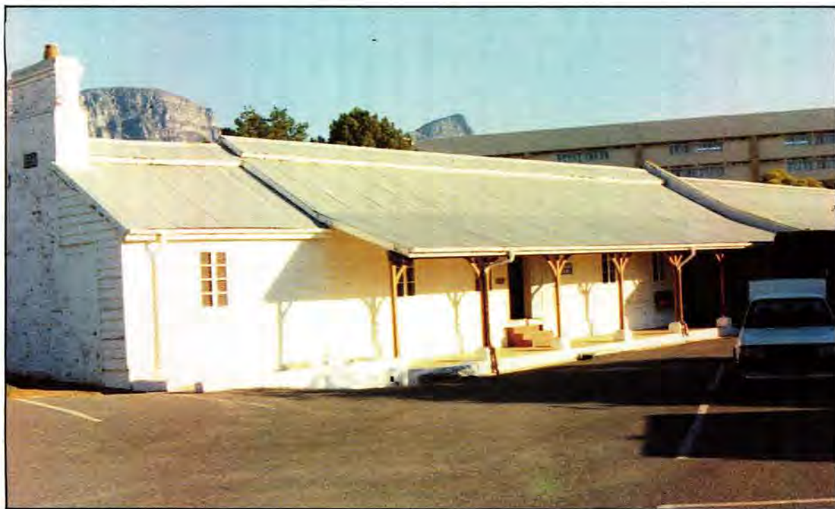
This wood and iron bungalow housed the CPGI shop in Wynberg from 1921 until 1961. It was taken over from the Imperial authorities in that year and might well have housed the SAGI canteen from before the First World War.
