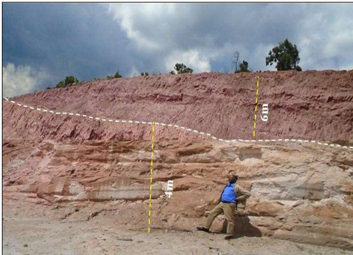
Figure 3. Section view of the open pit with the overburden material (top) and kaolin ore (bottom).
