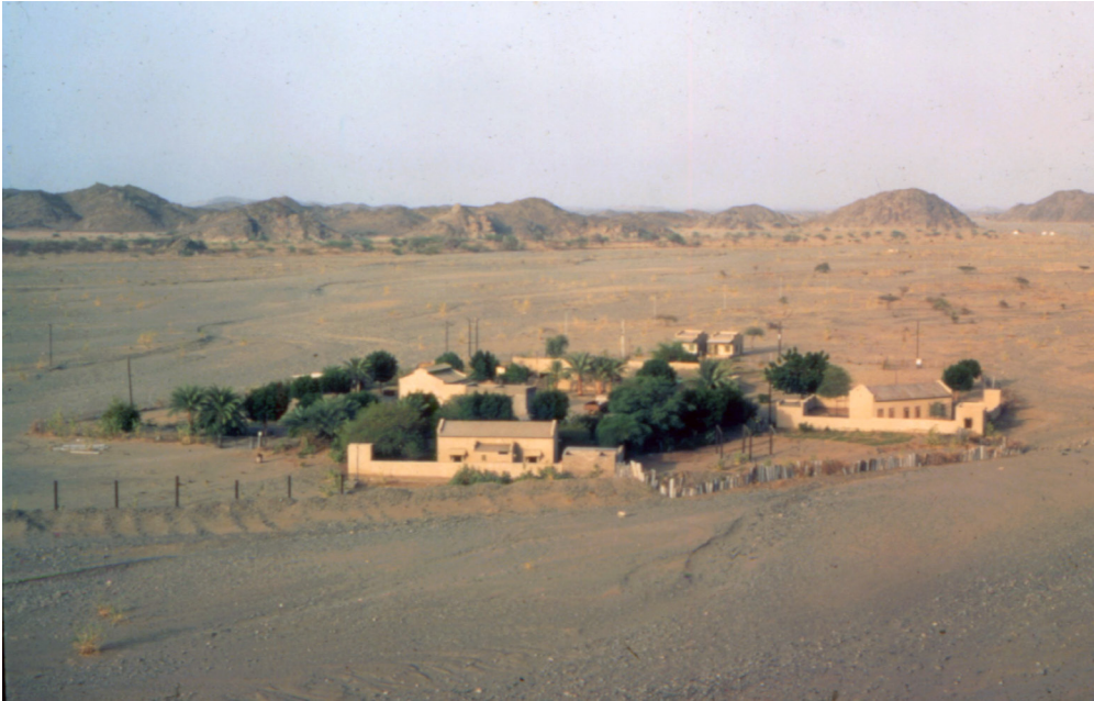
Figure 1. The Khor Arba'at water pump station in September 1984.
