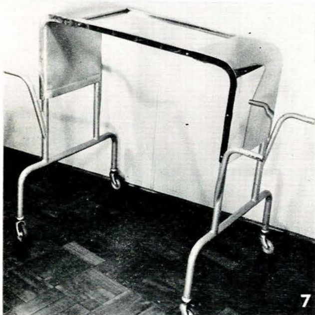
Fig. 7. Overbed table incorporating lead shielding.
