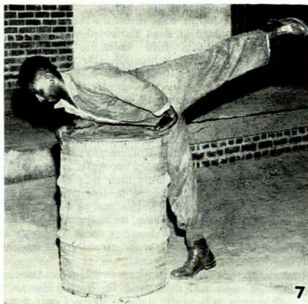
Fig. 7. The use of body weight in lowering a drum.
