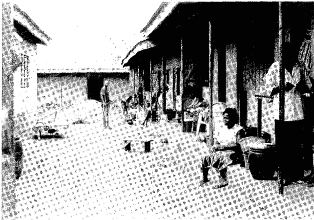
Fig. 2A. A typical TBS centre located at Afuze in Owan East Local Government Area of Edo State, Nigeria. The centre was built to accommodate the TBS's family, patients and their relatives. There are 25 rooms, each of which accommodates 3 patients with their relatives.
