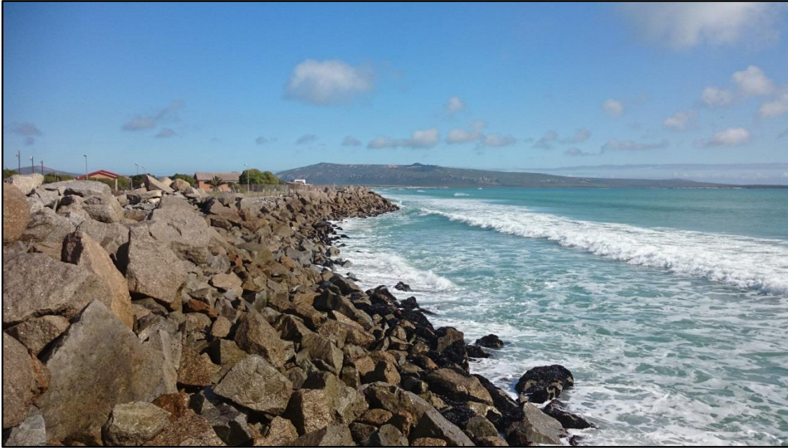
Figure 8: A photograph of a part of the breakwater that was constructed during the 2002 in order to stabilize beaches in and near Langebaan.
