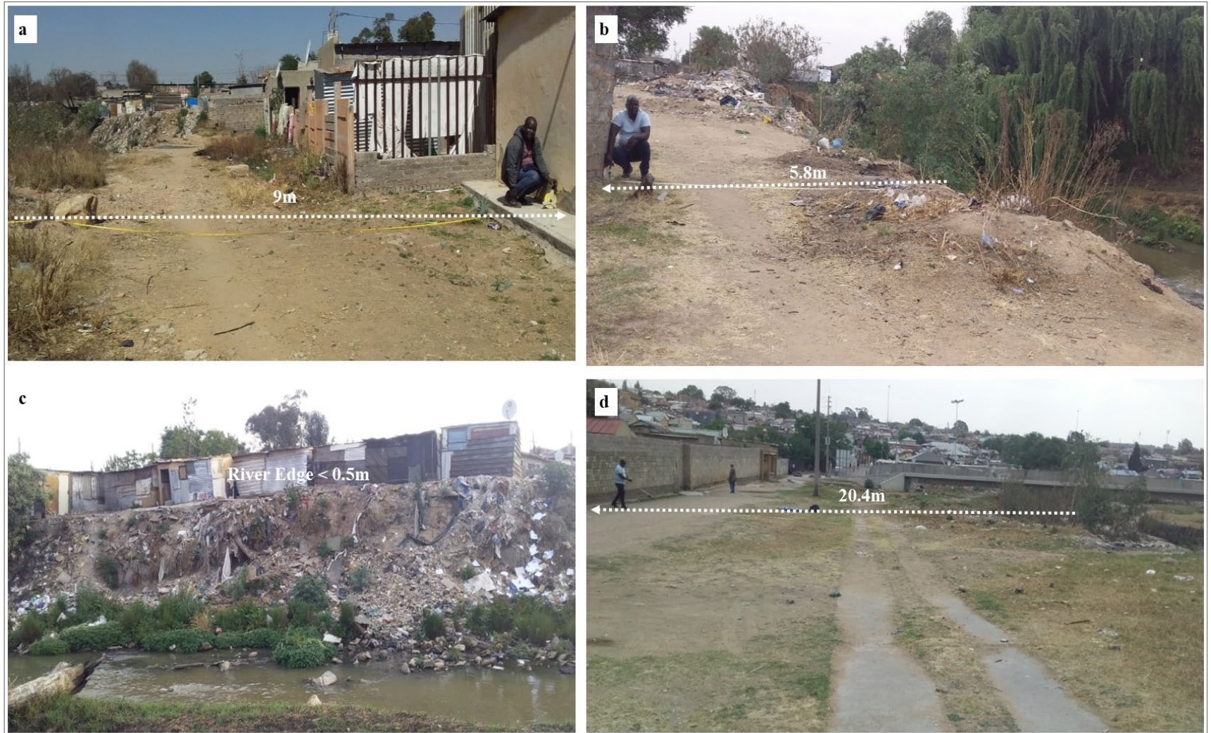
Figure 10: Proximity of residential buildings from the riverbank
