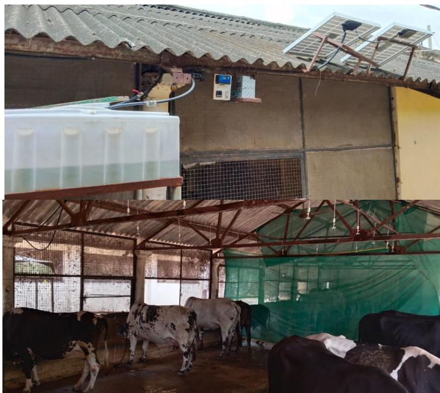
**Figure 1.** Solar power-assisted cooling system in an animal housing structure
