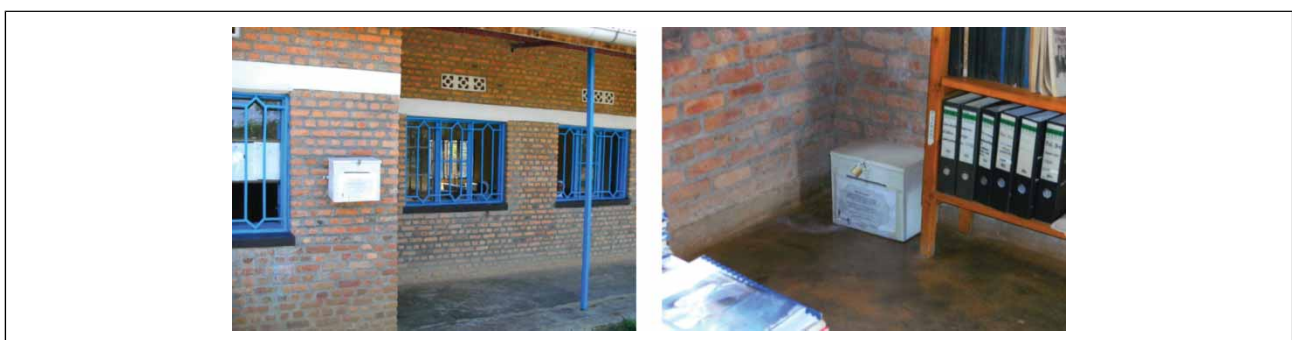
Fig. 1. The left image shows a mail box that is correctly installed, the right image is an example of a mail box on the school library floor.
