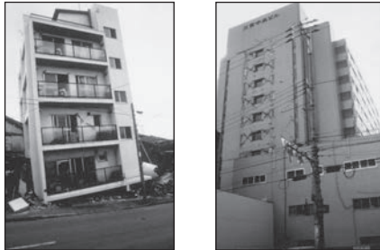
FIGURE 3 (above left). Typical example of building class #8 consisting of ‘reinforced concrete shear wall, without moment resisting frame, medium rise’. Source: EMS98 (op. cit.)
