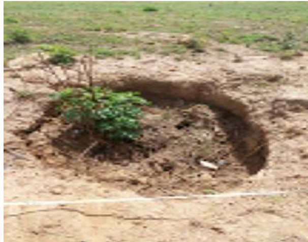
Figure 12: Sinkhole within the premises of the Church property
