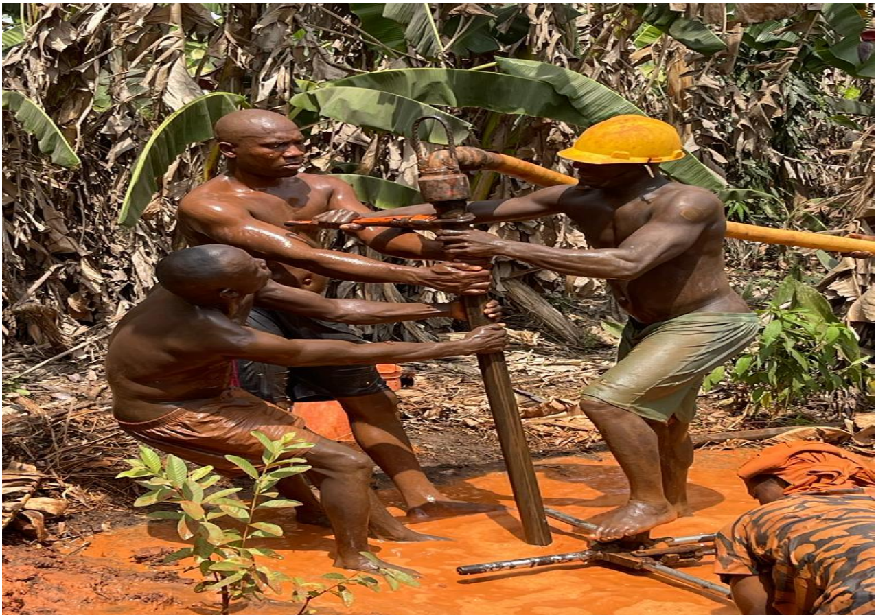
Figure 3: In operation of the borehole drilling in the field in site 1
