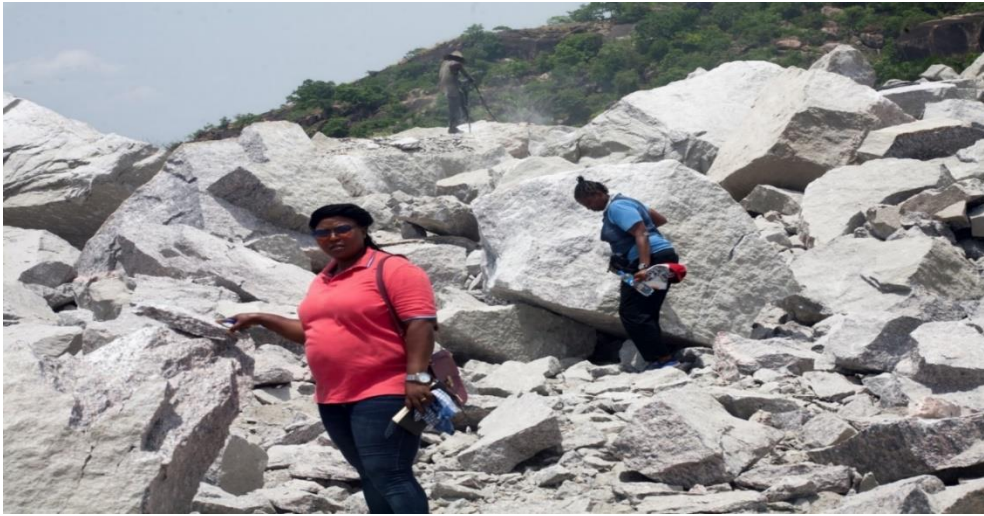
Plate 5: Field Photograph showing a driller on top, these granite boulders will require re-blasting before transporting to crushing plant at a quarry in Kporoko Village, Nigeria (site No. 2)
