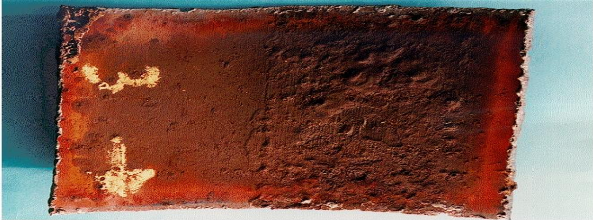
Fig. 1: Internal corrosion of a crude oil pipeline
