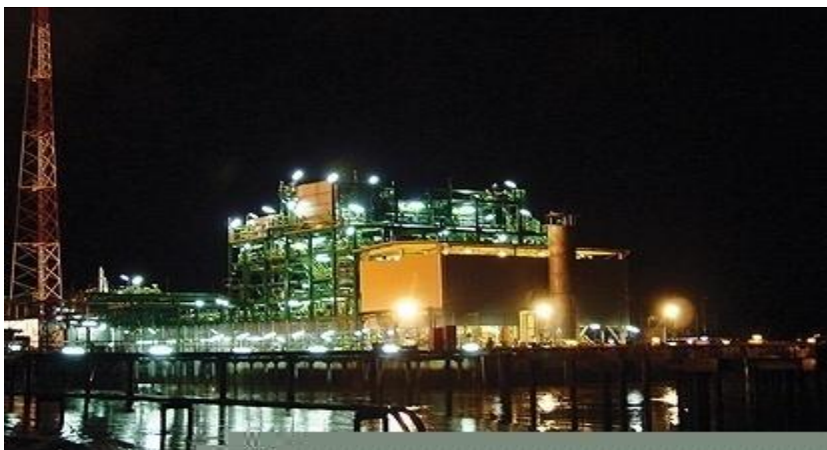
Figure 2: The Cawthorne Gas Channelling has been helping to eliminate flaring in Nigeria by recovering 200 million standard cubic feet per day of associated gas from oil fields. (Source: http://www.sustainability.mottmac.com )
