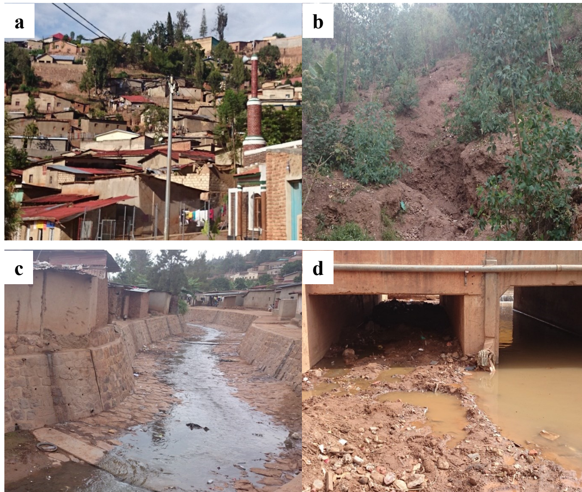
Figure 2: Field photographs from the study catchment: a) Informal settlements on steep slope; b) Poor vegetation cover; c) Illegal occupation in flood risk areas along the riverbank; d) Location of the study catchment outlet.
