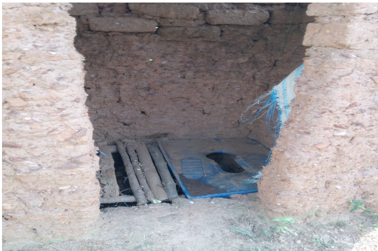
Figure 4. 2. The urine diversion pit latrines using Ecosan slabs received from UNICEF 2015 in Gahunga Sector.
