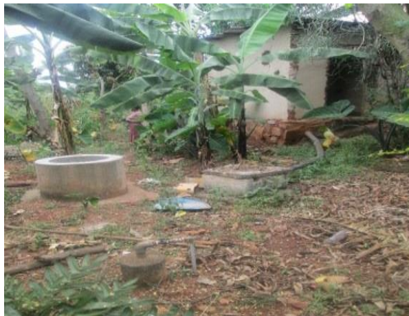
Picture 1: Household Biogas plant connected to toilet
