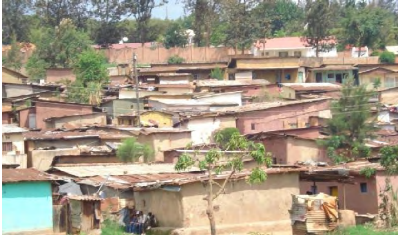
Figure 2: Informal settlement in Muhima Sector Source: Taken by Author in September 2009
