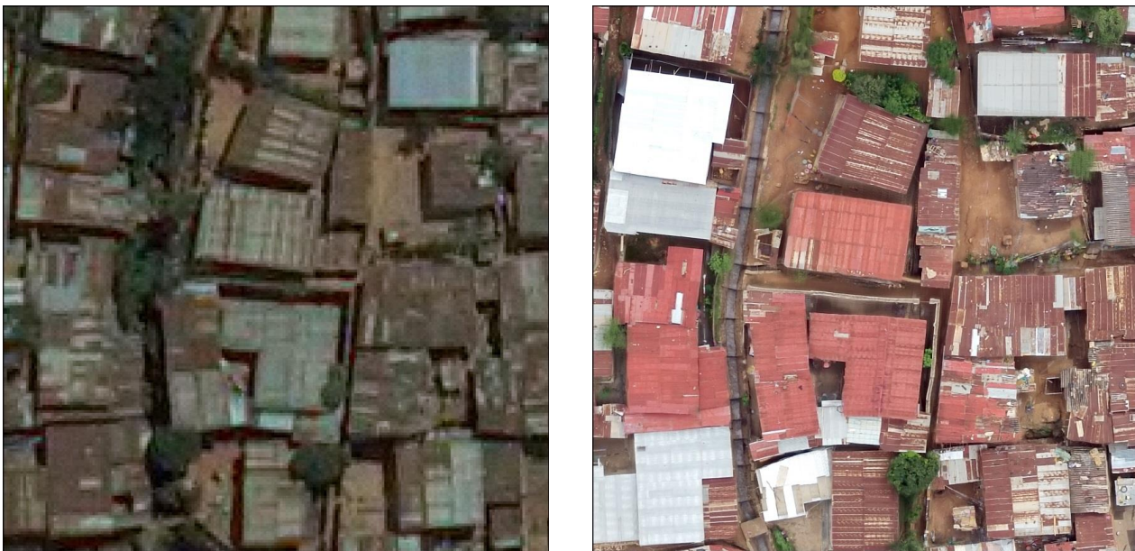
Figure 4: The added value of the UAV data is clearly visible when comparing the information provided by the 2008 orthomosaic (left) to the 2015 UAV orthomosaic (right). Note the enhanced visibility of objects in the scene as well as the appearance of new structures.
