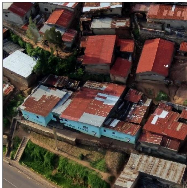
Figure 3: Sample of the 3D model (mesh) obtained from the UAV data over the project area.
