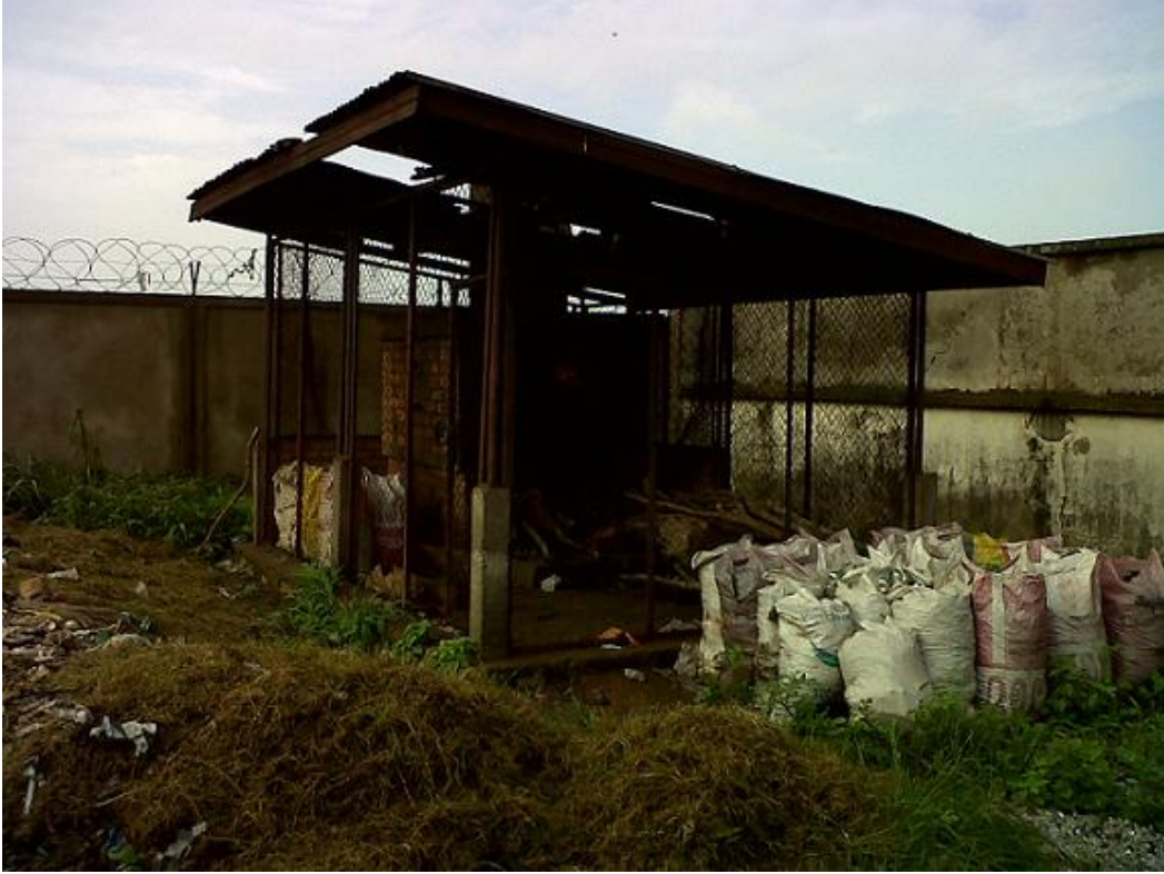
Figure 7: Montfort type of incinerator at the laboratory of community hospital is an old inefficient incinerator, with significant smoke during waste disposal
