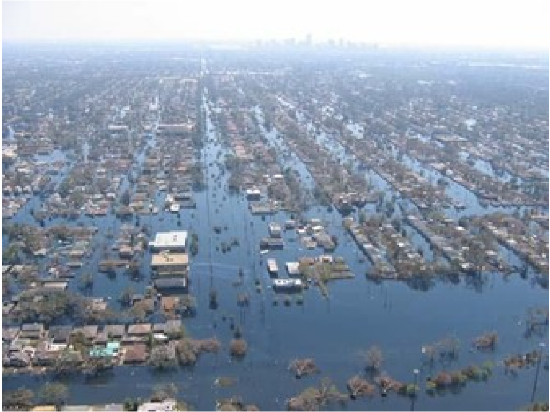
Figure 9: Hurricane Katrina damage (Source: NWS/Lieut. Commander Mark Moran, NOAA Corps, NMAO/AOC)
