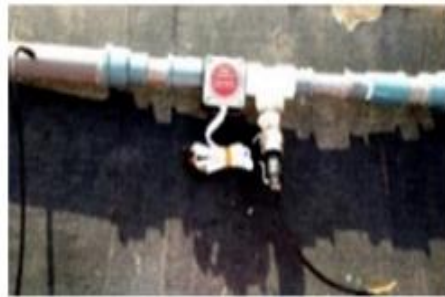
Figure 7b: Sensors installation
