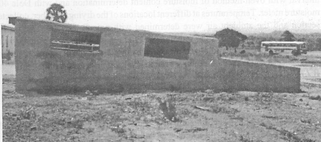
Plate 2: Side View Of Mud Type Solar Crop Dryer At New-wuse Village (Niger State)
